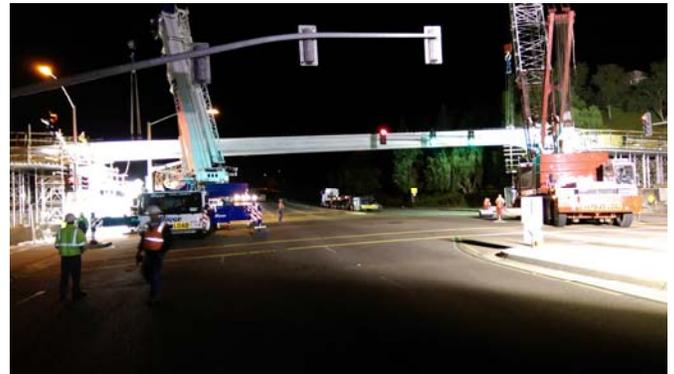
*Construction crews install girders for Shoal Creek Pedestrian Bridge.*
